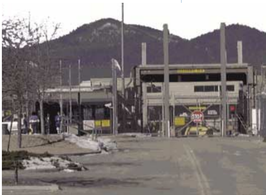
The entrance to the TA-55 Plutonium Facility.
